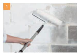
Applying 1 coat of *Dulux Texture Primer*<sup>™</sup> is recommended to condition the surface and aid application of successive coats. Areas that aren't accessible by roller, should be cut in with a brush.
