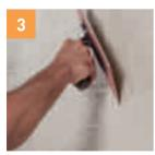
Levelling must continue before the skin dries. Working from the ground upwards, hold the plastic float against the surface so that the leading edge is raised and angled at approximately 45 degrees. This process can be done in pairs, with one person levelling as the other continues delivering product to the wall. Push the material across the surface to fill joints and low spots. This process should broadly distribute and level the roller applied texture before it sets.
