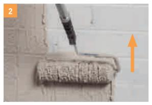
Applying 1 coat of *Dulux Texture Primer*<sup>™</sup> is recommended to condition the surface and aid application of successive coats. Areas that aren't accessible by roller, should be cut in with a brush. Apply 1 coat of *Dulux Texture Primer* with a roller and allow 4 hours dry time before applying *Dulux Texture Full Cover Roll On*.
